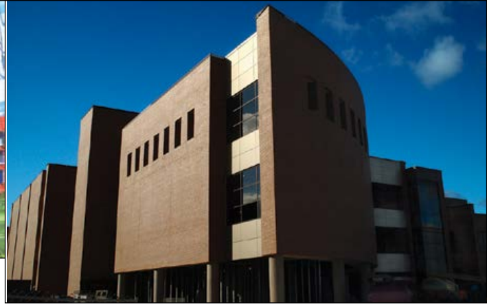
The new building for the B. Thomas Golisano College of Computing and Information Sciences is expected to open in spring 2003.
