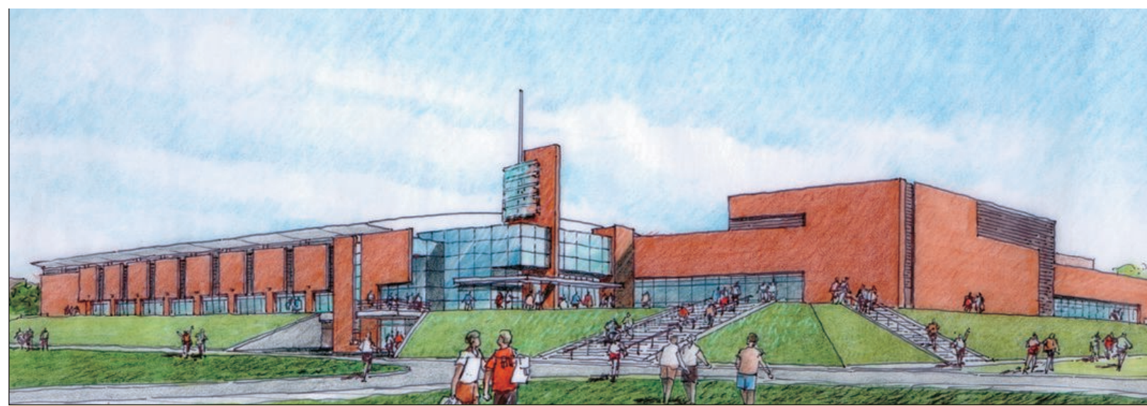
RIT's Field House and Activities Center, to be built adjacent to the Hale-Andrews Student Life Center, will be a multi-purpose facility for recreation, athletics and other campus activities.
