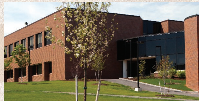
Heidelberg printing facility, Louise M. Slaughter Building
