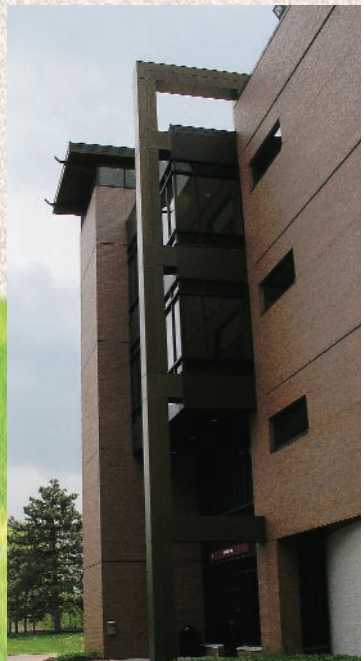
ell Building addition
