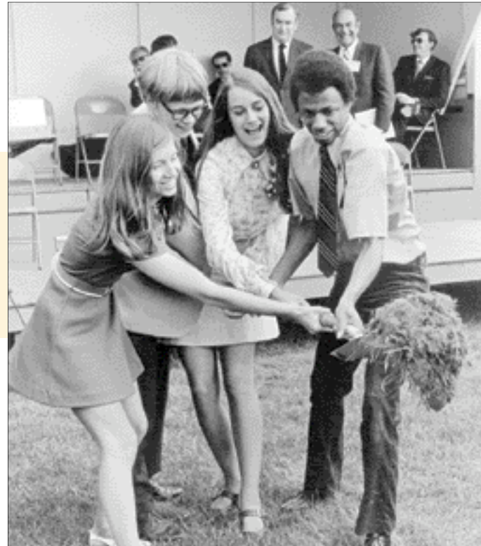
Ground was broken on June 4, 1971, for construction of the NTID complex. Four students participated, from left: Linda Kessler '73, Thomas Tyberg '71, Barbara Kowalczyk '73 and Charles Jones '73.
