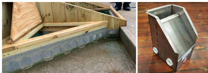
Image 4 (LEFT): Double-layered chicken wire filtering out clippings as water flows through trough. Image 5 (RIGHT): An example of a pre-fabricated separator—a hydroscreen—to filter out clippings. A bucket can be placed under this device to collect filtered clippings.
