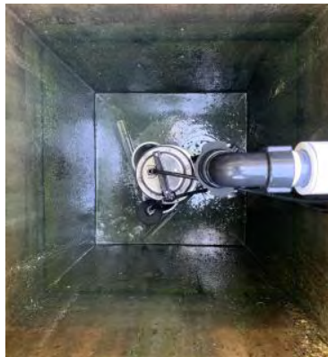
Image 11 (LEFT): A sump pump installed at bottom of well Image 12 (RIGHT): Dispersal of water into the settling tank using PVC pipe with holes drilled in the bottom
