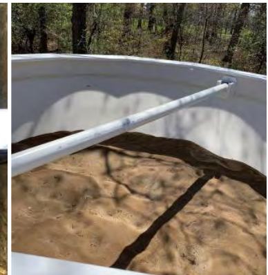
Image 11 (LEFT): A sump pump installed at bottom of well Image 12 (RIGHT): Dispersal of water into the settling tank using PVC pipe with holes drilled in the bottom
