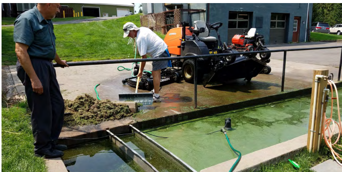
Image 7: Clippings buildup at initial screen
