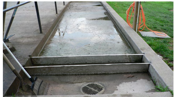
Image 6: A pad feeding a trough with two screens to filter out clippings
