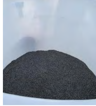
Image 14: Gravel base layer
