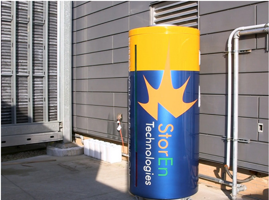
StorEn VFB Battery
