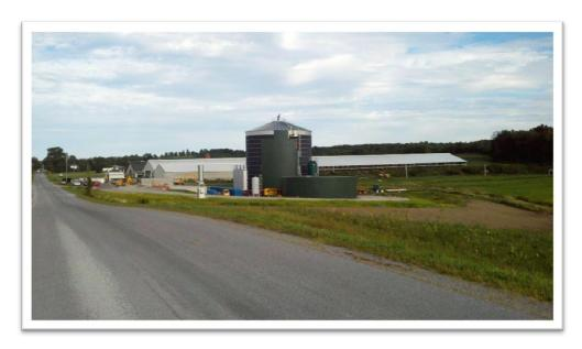
Synergy Anaerobic Digester processes 100,000 gallons per day of manure, food grade and organic waste.
