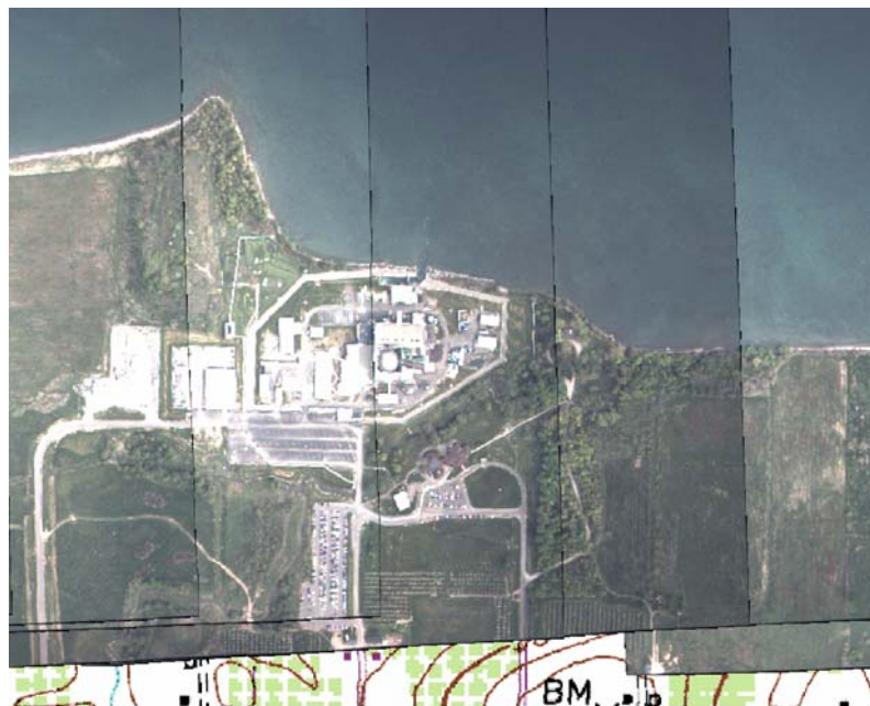
Figure 3.5.2-1: Realtime image of nuclear power plant overlaid on USGS map
