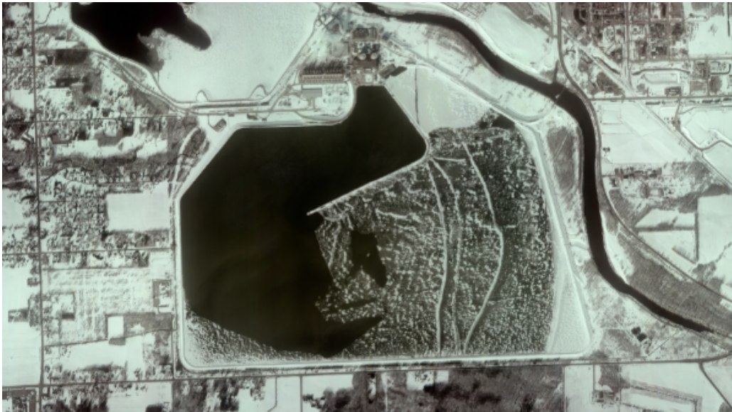
Figure 3.13-19: Midland Cogeneration Venture power plant in Midland, MI. This gas-fired power plant receives cooling water from and discharges to a closed cooling lake originally designed to support cooling of a planned nuclear plant at this site. Due to the oversized nature of this lake, it does partially freeze during the winter months.
