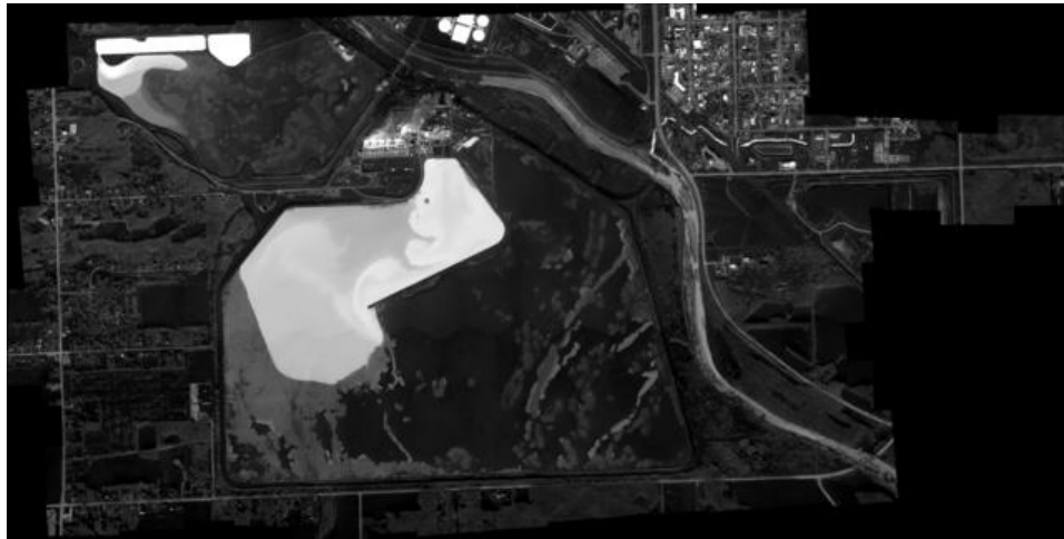
Figure 3.8-17: Longwave infrared image mosaic of the Midland Cogeneration Venture power plant in Midland, MI. This image was collected on January 26, 2009 at an altitude of 3,000 ft using the RIT WASP sensing system.
