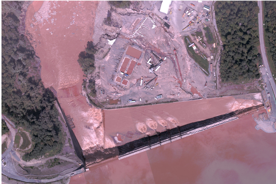
Figure 3.10-30: : Flood waters pour over the Gilboa Dam on Schoharie Creek following rains from Irene. Imagery provided to NYS by IPLER with 4 hours after collection.
