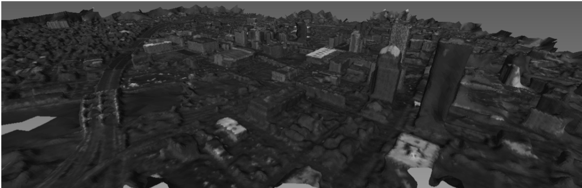
Figure 3.23-53: A rough form 3D "object model", extracted from the image-derived 3D point clouds, or x,y,z points. These buildings can now be cleaned and exported as a proper 3D city model.
