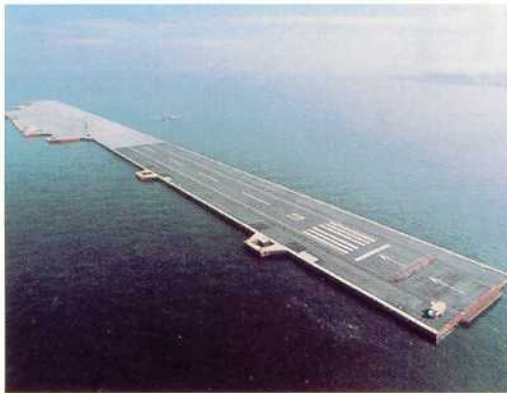
Mega-floats, developed with funding from The Nippon Foundation, are an environmentally friendly, inexpensive alternative to land-reclamation.
