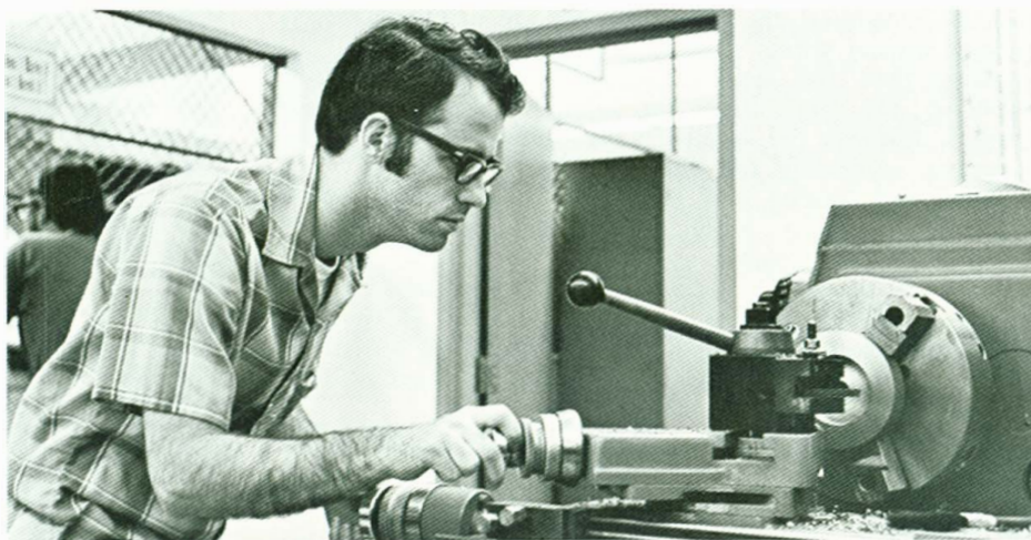
SPEED LATHE — Instructor George McCoy (right) explains to NTID student James Sweeney of South Hadley Falls, Mass. how to operate a Hardinge Speed Lathe.
