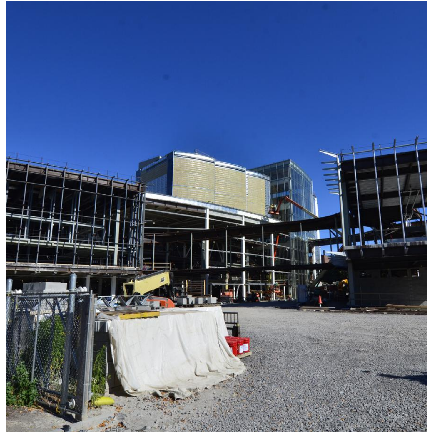
The SHED under construction
