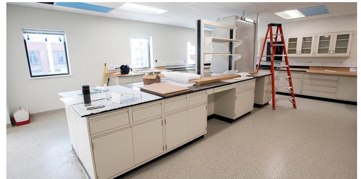
Brown Hall Renovation Interior in Process
