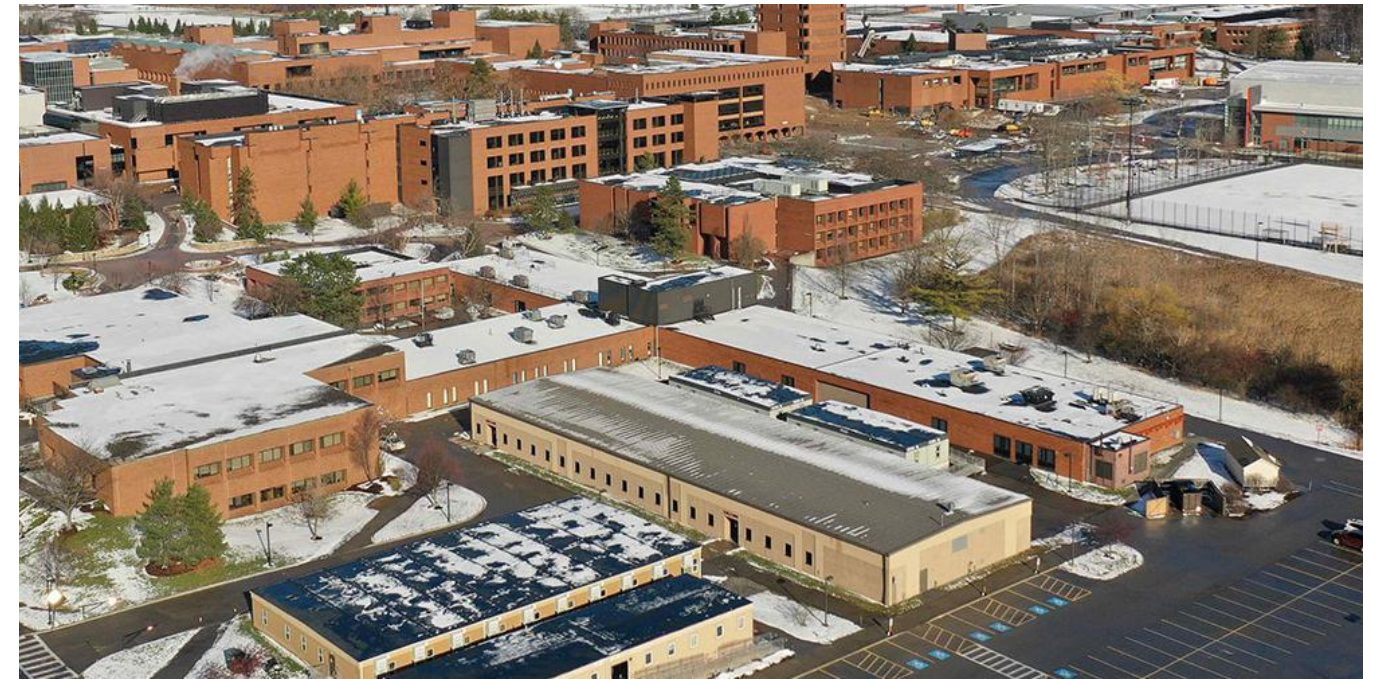
Brown Hall Renovation
