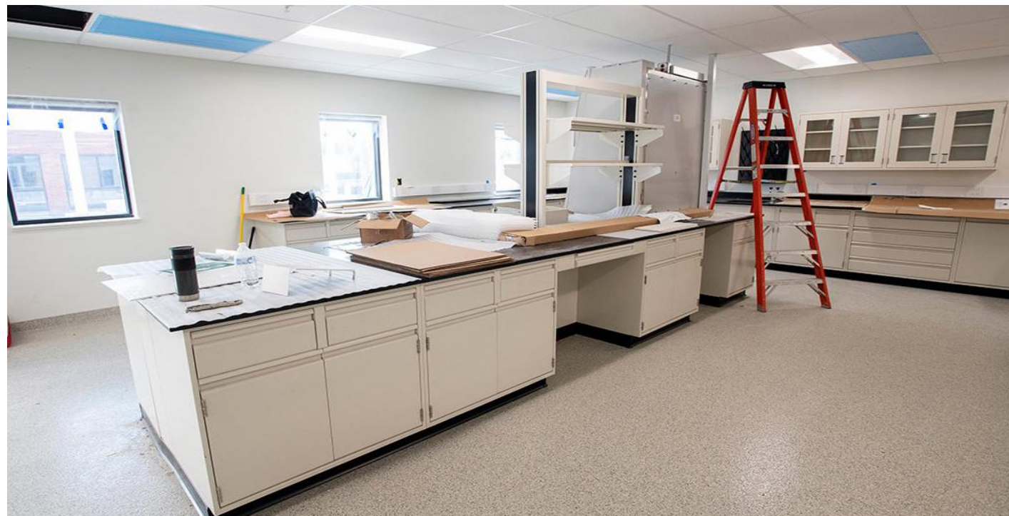
Follow the Brown Hall renovation for examples of flexibility
