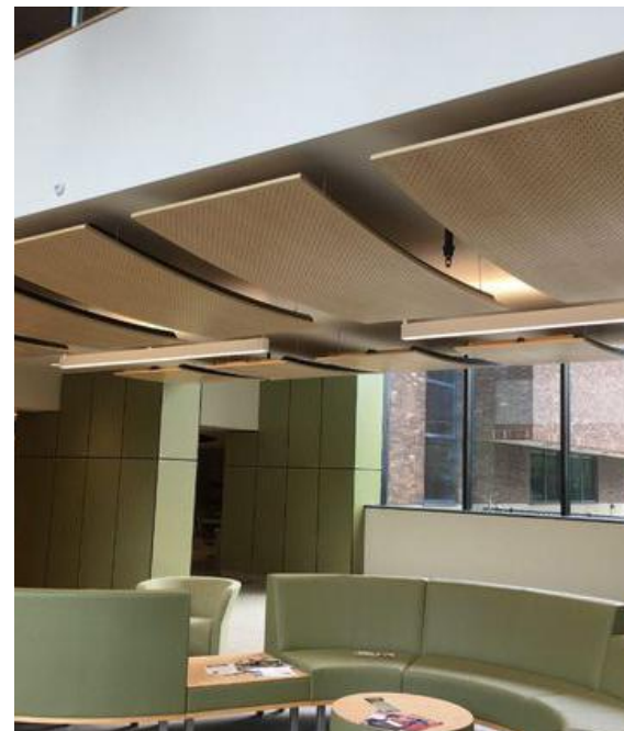
Acoustic Control Panels
