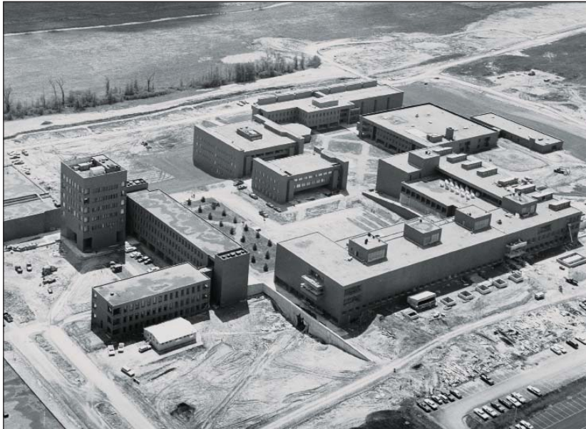
An aerial view of the campus as construction neared completion in 1968.
